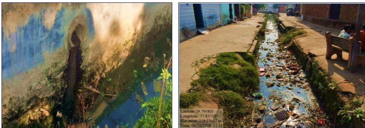
Fig. 3.4: Sewage and garbage disposal in Gadarjudda minor
