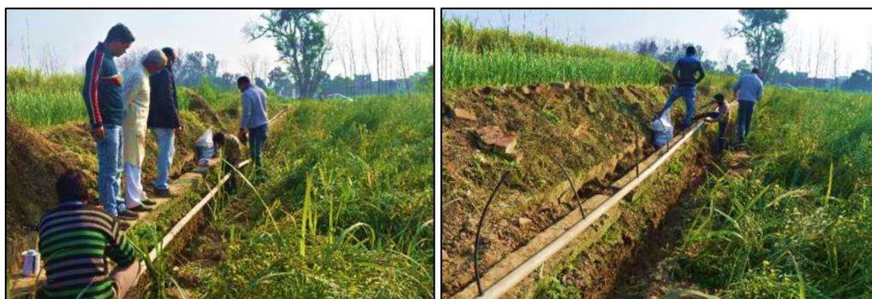
Fig. 6.1: Installation of micro-irrigation system
