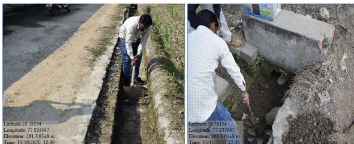
Fig. 1: Cleaning of the watercourse
