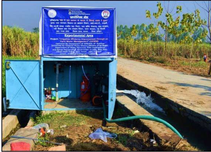
Fig. 6.2: Head unit of micro-irrigation system
